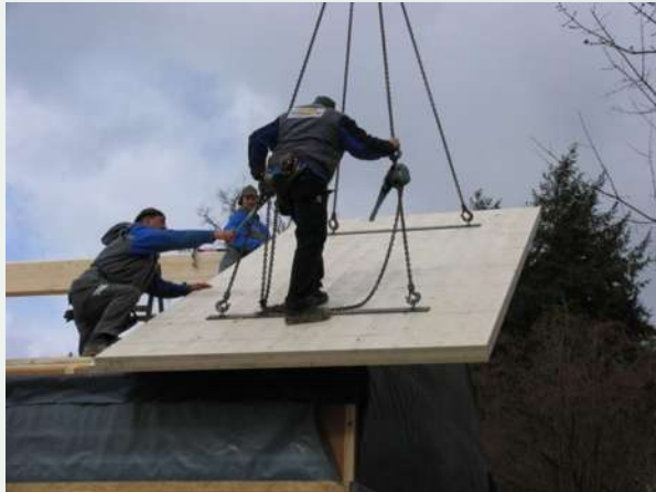
assembling of roof elements
