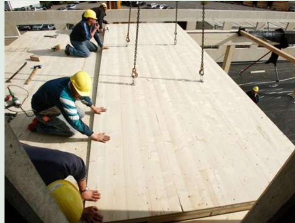
assembling of ceiling elements
