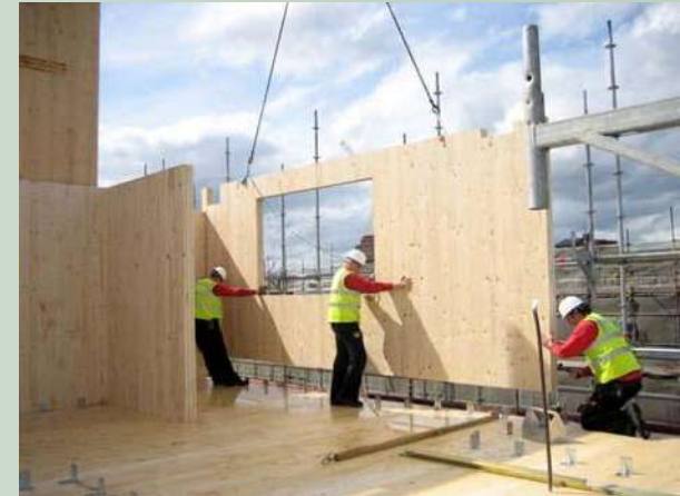
assembling of wall elements
